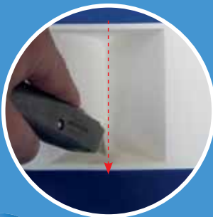
Cut along the centre-marking.
