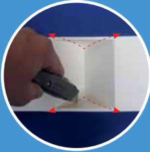
Cut only along the marking.
